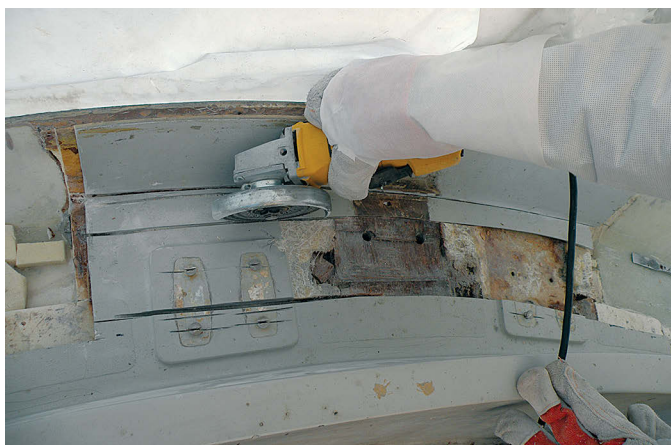
Because of the way the deck was joined to the hull, Steve had to cut into the bulwark, at left. The deck skin also had to be cut out to expose the saturated balsa core. Mary removed the rotten core with hammer and chisel, at right. The white hose is part of the dust collection system.
