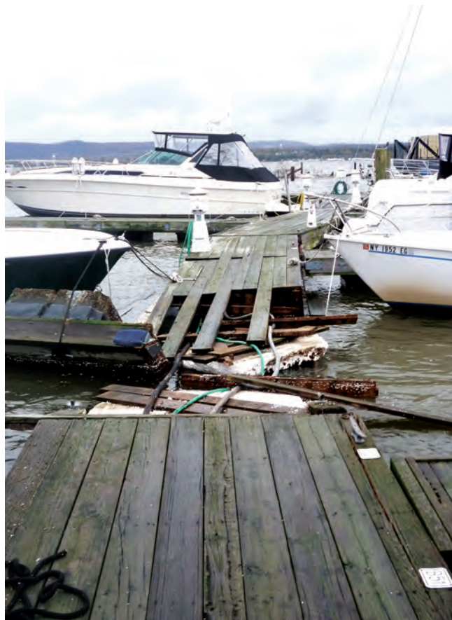
In the marina, docks broke loose when they were lifted above their pilings, above, but the boats attached to them in general fared quite well and suffered little damage. An assortment of debris lodged in the boatyard fence, below, shows the height the water reached.
