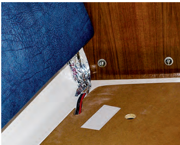
Running the heavy-duty electric cable from the battery to the windlass presented a challenge.
