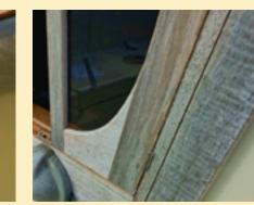
The gray glazing tape is barely visible through the smoked polycarbonate on the inside of the door, at left, and not at all visible from the outside, at right.
