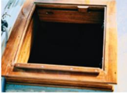
clamped the wood in place and transferred the shape with a pencil and a scribing block.
