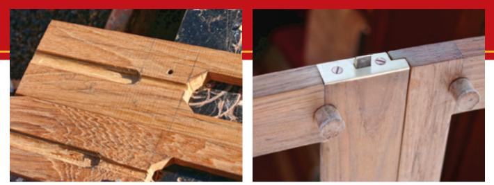
Benjy made the center door stile in two pieces and, with a router, cut grooves in them to take the homemade latches and controls, at left. The wooden plugs with leathered ends prevent the doors from bending when leaned against, at right.
