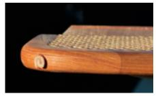
Benjy wanted his companionway steps to work harder so, starting with a mockup, opposite page at bottom, he built a box that was steps, a seat, and a trash receptacle, below. Leather, rolled up and glued into a hole, softens impacts with the head door, above.
