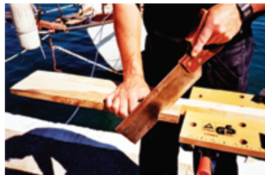
After planing down the shaft, Richard made a cut to form the shoulder of the blade.
