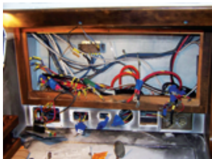
Because acidic smoke residues could cause problems down the line, the electrical panel, at left, had to be removed, cleaned, and rewired, at right.
