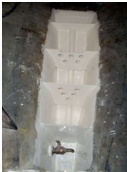
Coating the sides and bottom of the tank.
