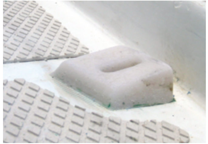
Cleaned up and sanded, the island has become part of the deck.
