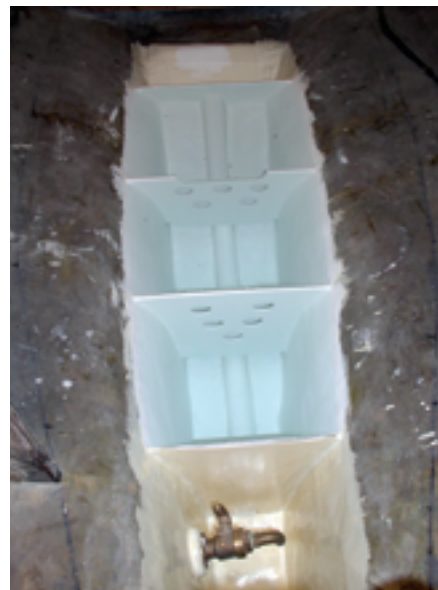
Testing for watertight integrity.
