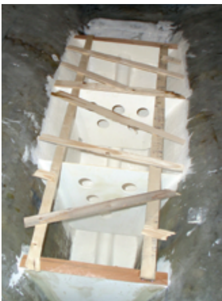
Making the template for the tank top.
