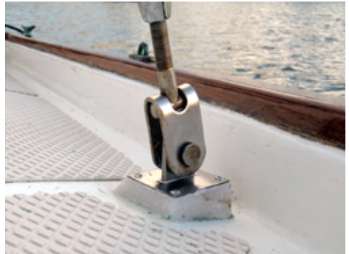
Once leak-prone, the chainplate is now high and dry.
