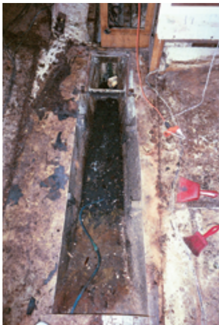
The old tank removed, the bilge awaits a cleanup and a new role.
