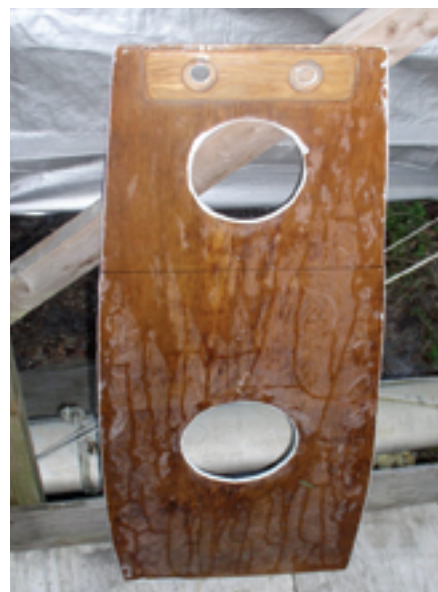
Cutting inspection ports.
