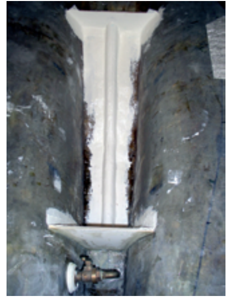
Glassing in the forward and aft bulkheads.
