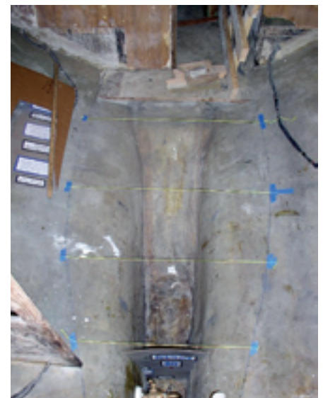
Marking out for the bulkheads and baffles.
