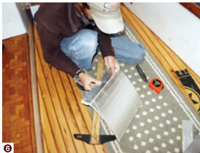
The aft cabin before the insulation treatment, (5). Dave snaps the Celotex to form a curved shape, (6).
