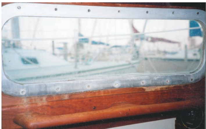
Leaks from the Tartan's ports had stained the interior teak and corroded the inner frame.
