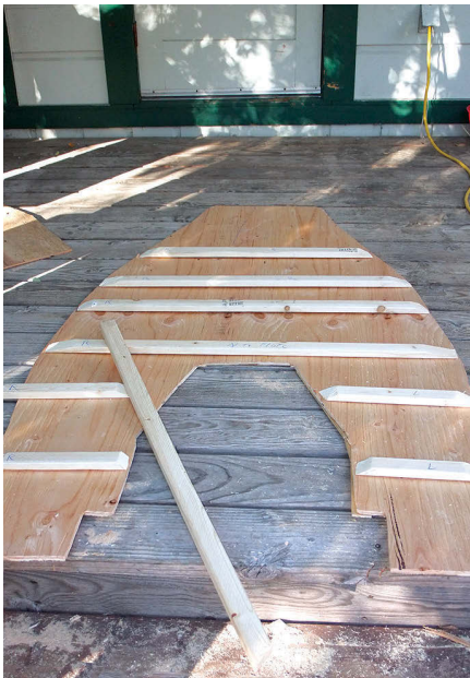
A friend made a floor for the dinghy, at left and above left, and a seat. After repairing the holes, Robert painted the boat inside and out and fitted a gunwale guard of wood, foam, and fire hose. The result is a serviceable rowboat with a new lease on life, at right.
