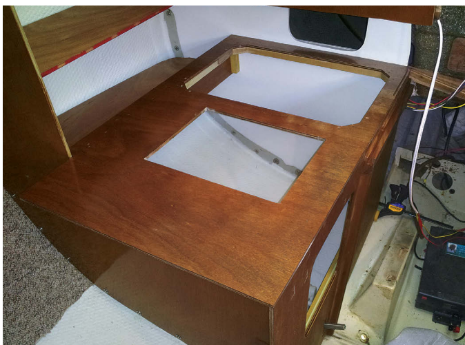
Ric sealed the countertop with penetrating epoxy, above left, then epoxied Formica to it, above right. The countertop and front are not yet installed. He fitted the Engel into the countertop hole, built out the lid supports, then eased the whole assembly into place, below.
