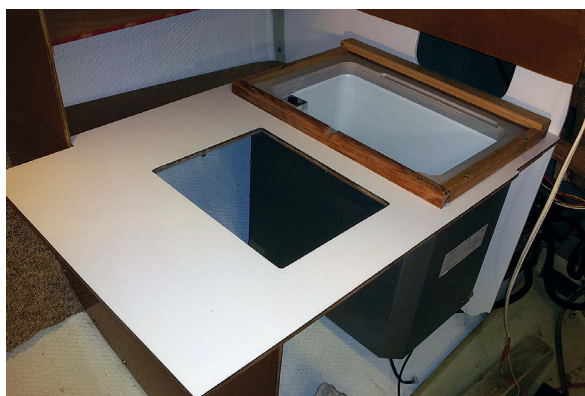
Ric sealed the countertop with penetrating epoxy, above left, then epoxied Formica to it, above right. The countertop and front are not yet installed. He fitted the Engel into the countertop hole, built out the lid supports, then eased the whole assembly into place, below.
