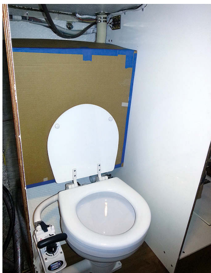
After gutting the head compartment, Ric fitted new bulkheads and a Marelon through-hull valve, at left. He made the cardboard mock-up for the tank after fitting the new head, at right.
