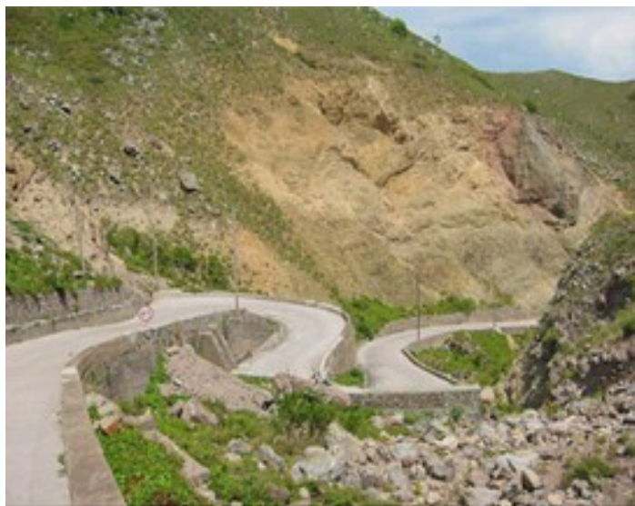
Saba switchbacks – Heading “up” to The Bottom
