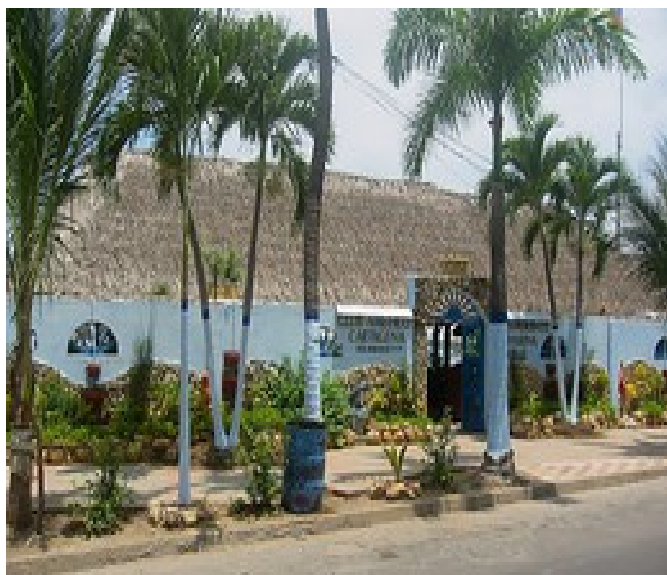
Club Náutico office, clubhouse and restaurant
