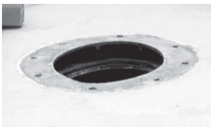
Clean partner area ready for epoxy fill.
