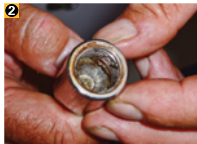
2 Inspect the female thread for signs of rust and traces of thread sealant.
