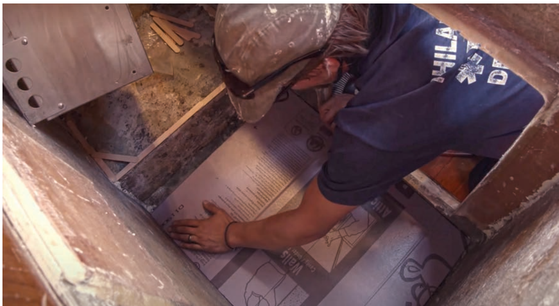
Positioning the Foamular XPS insulation in the bottom of the fridge compartment.
