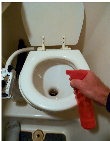
A spritz of holding-tank treatment before a final freshwater flush helps abate odors.
