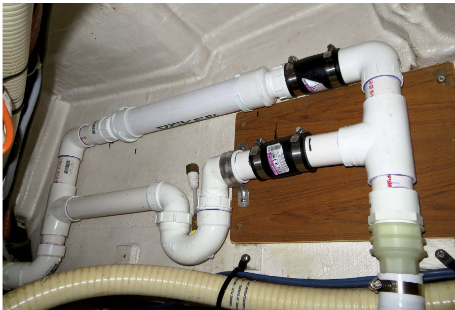
On his catamaran, Alan found a large-enough space to fit his vent system athwartships, where he also had access for checking the sight glass and changing the filter.
