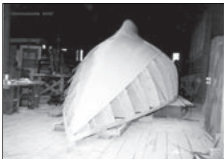
Building the plug for the mold of the Chinook, 1955, above.
