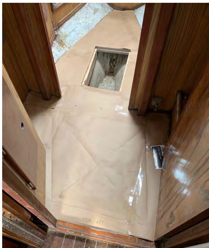
The template was traced onto the underlayment.
