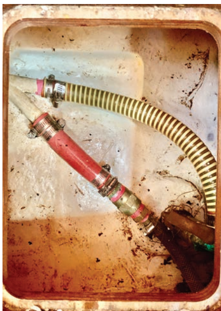
Left, a Y-fitting was run off the water intake.
