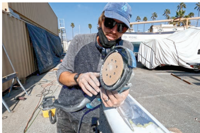
The author's husband, Chris, uses an angle grinder with a 5-inch hook-and-loop sanding pad to remove the mast's old paint.
