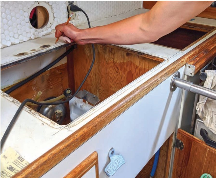
At left, Scott marks the cut and drill locations for the new faucet.
