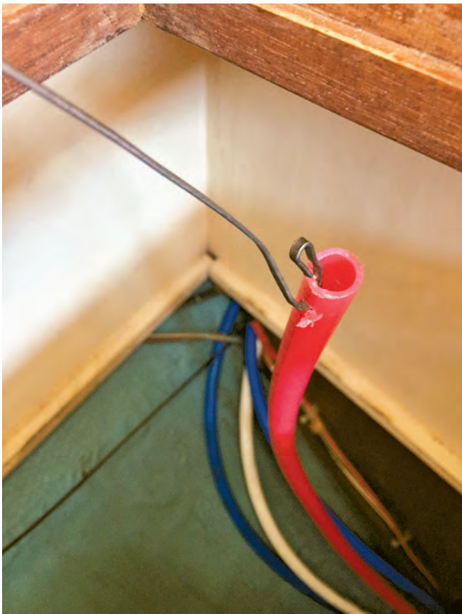
Electrician's fish tape, attached via a small hole in the end of the PEX line, made simple work of snaking the pipe through hard-to-reach areas.
