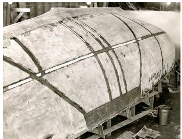
Balsa core applied to the inside skin on a hull plug. Note the areas of core removed to allow installation of solid fiberglass “strapping,” a technique eliminated in all subsequent cored construction at C&C. Credit Mark Bruckmann.
