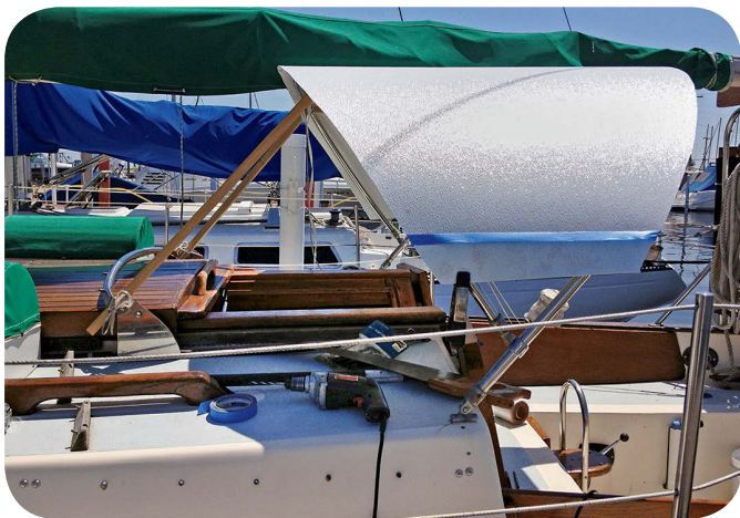
Charles cut the FRP sheet a little over size, at left, so he could play with the height of the dodger and the width of the hardtop. He also adjusted the height of the frame, at right, to balance the sight lines forward with ease of access into the companionway.
