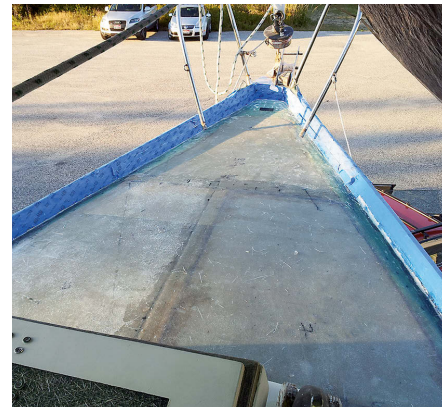
Before recoring the foredeck, Jon took measurements of the hardware locations, far left. He cut out a section of the top skin and chipped away the old core, at left, cleaned up the area, then laid the new core and the first layer of fiberglass, above.
