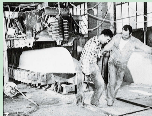
In the mid-1940s, Taylor Winner built runabouts using a rubber bladder male mold, a metal female mold, and heat to cure the resin, center and above.
