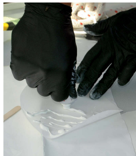
Chafe damage, at top of page, is a good candidate for a 5200 repair. Cut a patch to overlap the damaged area and wipe it and the sail with acetone, at left. Apply the 5200, at right.
