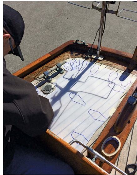
Shipwright Peter Taprell traced the deck edge onto Mylar, at left. The Mylar doesn't have to be an exact fit because tracing around the "fish" establishes the perimeter of the deck with precision, center. The finished tracing of the aft starboard deck has lots of marks, at right.
