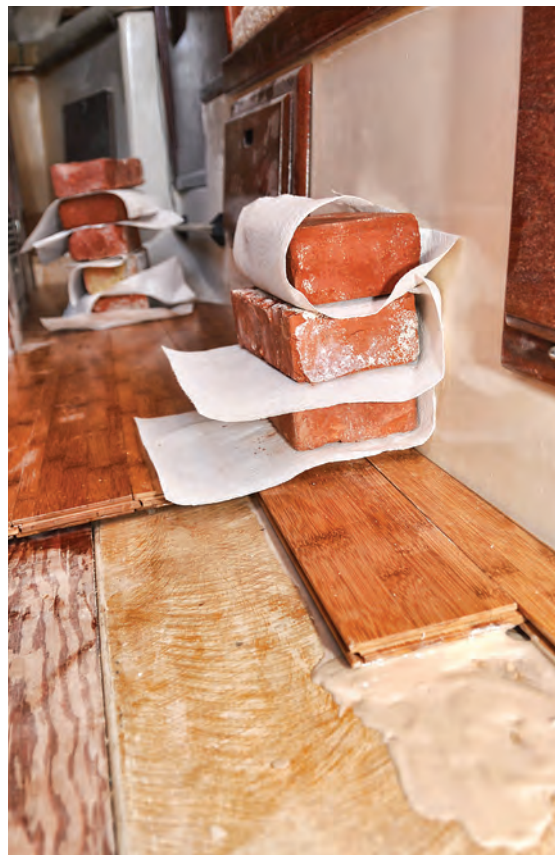
Working in tight quarters, Bill prepares to lay the sole next to the head compartment, at left. Bricks weigh down the boards while the epoxy sets, at right. Genie marks the boards after Bill has cut them to fit, below left. Bill applies epoxy to a board prior to setting it in place, below right.
