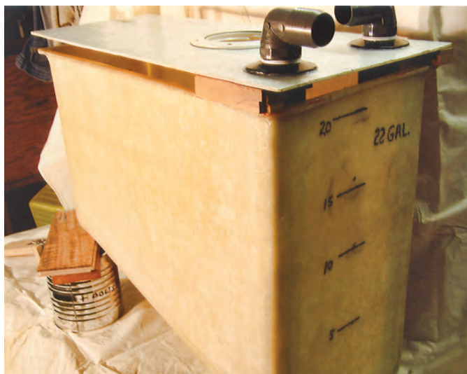
Almost there ... Ken has finished the tank and its top, marked the 5-gallon fill levels, and fitted the plumbing to the tank top.
