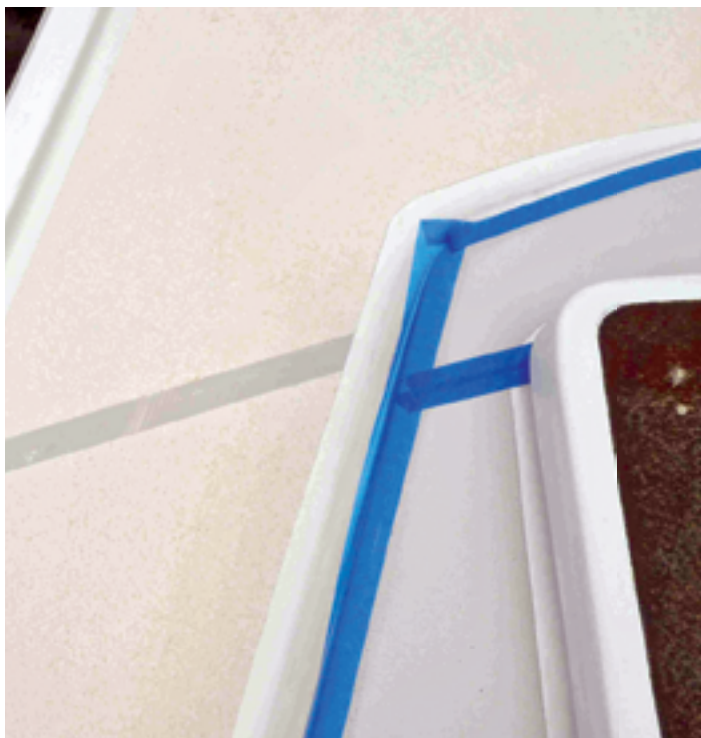
The borders have been painted and the tape laid out to mark the areas to receive KiwiGrip, above. Stephen divided large areas into more manageable smaller sections, below.
