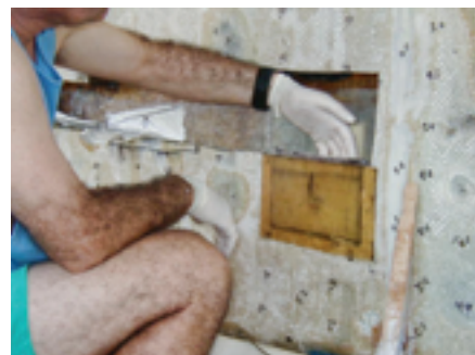
To prevent water from lingering in the bilge, Randy chiseled out a small sump to hold a pair of bilge pumps, at left. The rebuild began with fiberglass laid from the inside against a form, at right.
