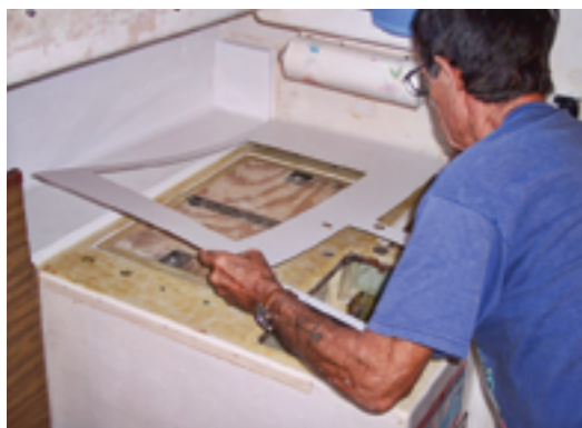
Bruce laid new Formica on his countertop, above. He fitted a shelf in the front to hold pots and pans, at right, and a space-saving towel rack on the face, at far right.
