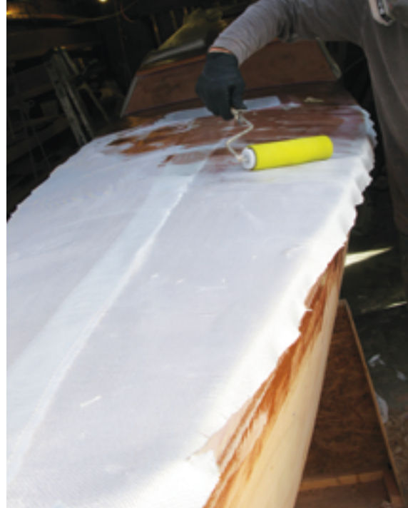
A coat of fiberglass cloth and epoxy will toughen the hulls' exteriors, above. Two hulls take over the driveway, below.
