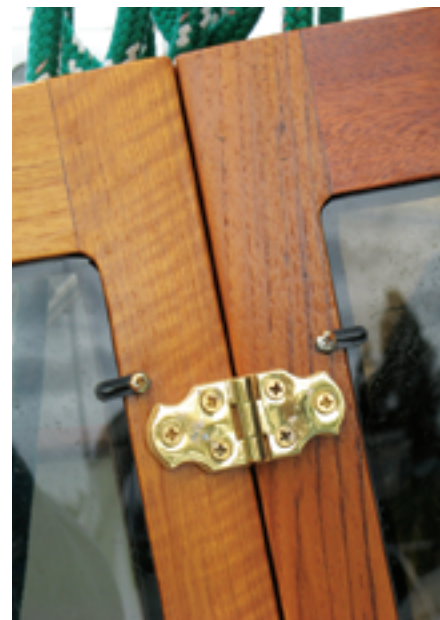
Gary fits the bi-fold doors onto the pintles that serve as hinges, at left. This view from the inside shows the brass hinges and the turn buttons that hold the inserts in place, at right.
