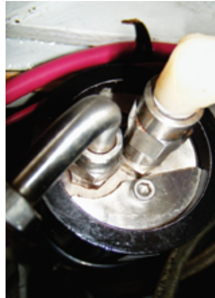
On this end cap of the pressure vessel are the inlet for high-pressure seawater (stainless steel) and the outlet for product water at low pressure (plastic).
