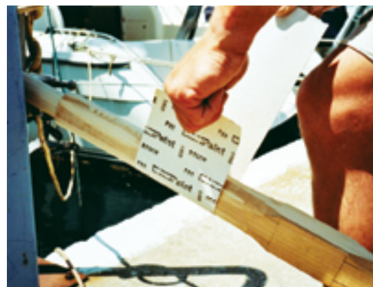
Sanding across the grain is an effective way to smooth a round object like an oar.
