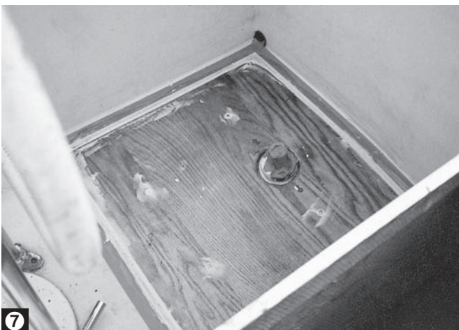
Reamer stuck in old bearing (1). Boring out the old bearing (2). Making the new bearing (3). Fitting the new bearing (4). Gaining access to wet plywood (5). Making the bearing support (6). New core installation (7). Putting the old floor back (8).
