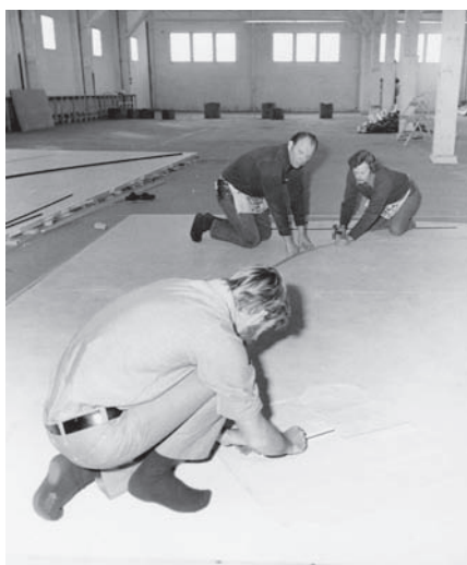
The original lofting of the 36's lines by Bob Wallstrom, John Perring, and Jim Marsh onto the Cabotcraft shop floor back in 1973.
