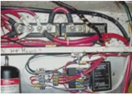
The wiring for the house battery for the solar cells, at left, and the engine battery wiring, at right.
