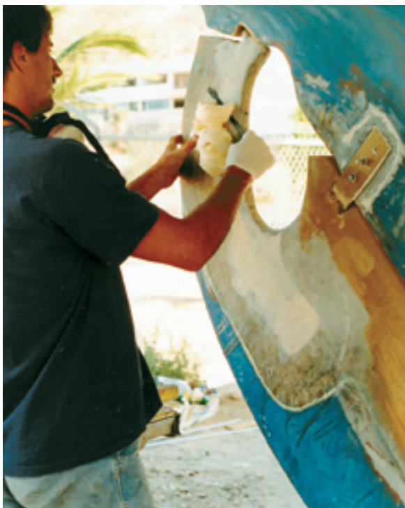
Sandy fills the large voids around the upper shaft with polyurethane insulation foam, above, before doing the final glassing and fairing at right.
