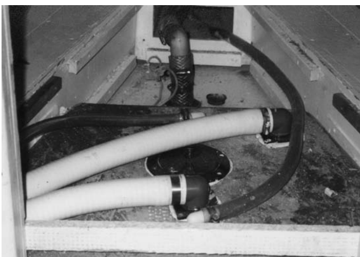
Finished tank installed with connections at the top.
