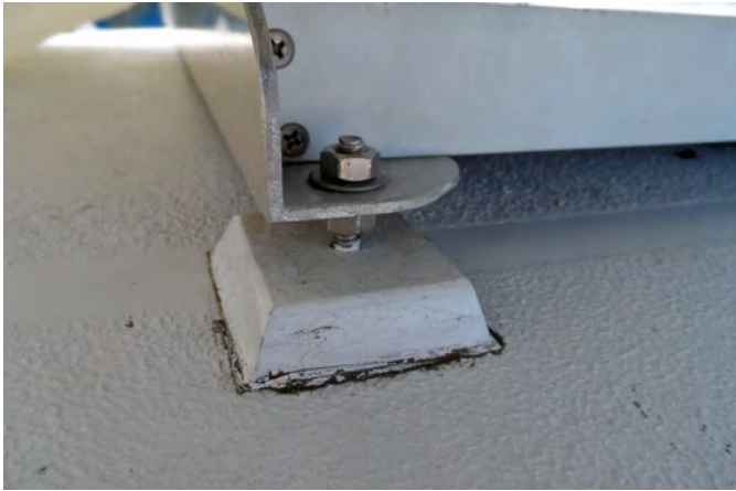
Drew used DIY Garolite studs to mount solar panels on his boat. Double nuts on the studs allow for accommodation of compound curvature and easy removal.
