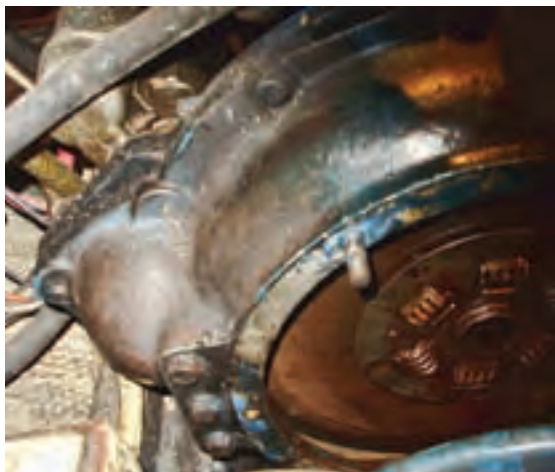
With the transmission slid back, the damper plate is visible inside the bell housing.
