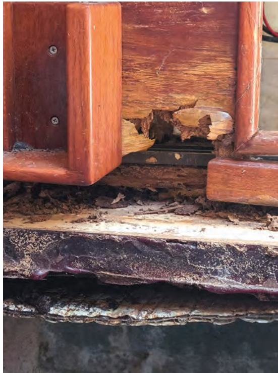
Left and far left, a close-up view of the galley damage.
