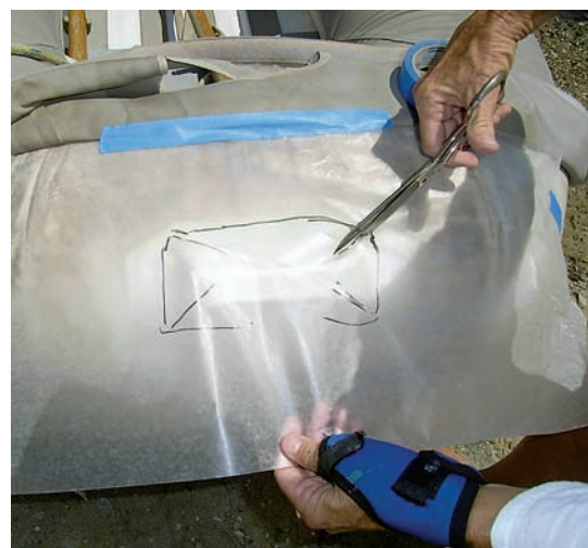
The first step in making a pattern is to mark the cutouts. Their initial outlines will only be approximate, since the clear-plastic pattern material is not flat when it is marked.
